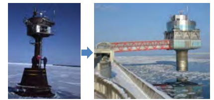
Fig. 5 Air-Sea-Ice Observation Tower (Left) changed to Okhotsk Tower (Right).
